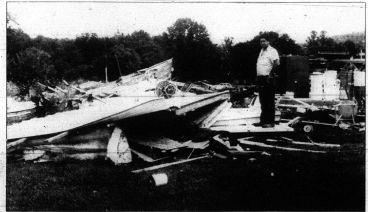
Eugene Philbeck stands amid the ruins of his garage and storage building that was destroyed by the high winds in Monday's storm. Philbeck lives on the Old Brodhead Road - (Photo by Raymond McClure.)
