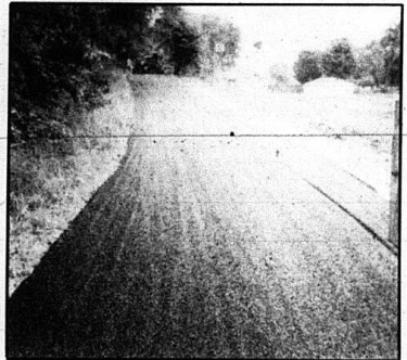
Kings Hollow Road looks different after the workmen complete their job.
