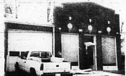
The Family Resource and Youth Services Centers are soon to be located in a renovated section of the old school bus garage building across the street from the Rockcastle County Board of Education.
