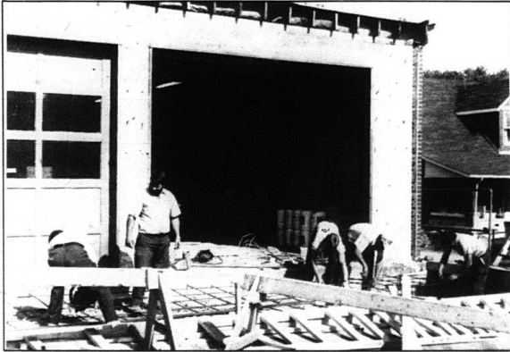
Mt. Vernon city employees are busy extending the fire department building to give firemen more room.
