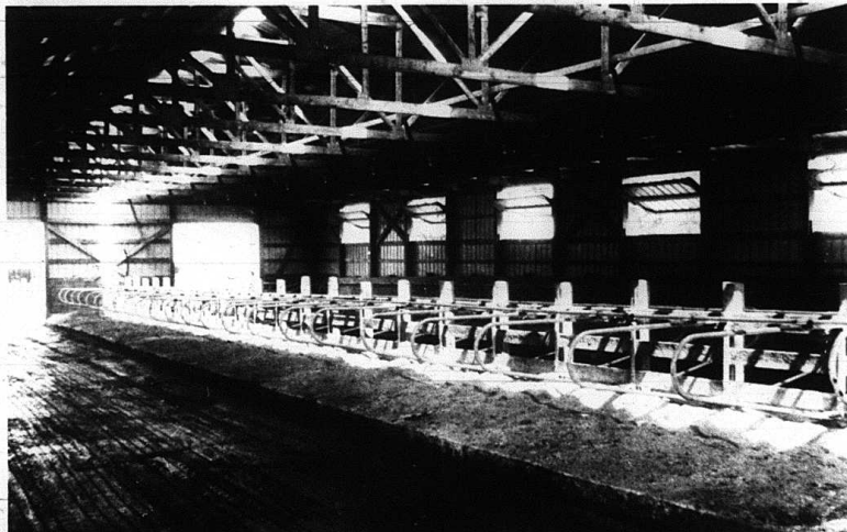
Hunt's major improvement is a feeding barn with a series of stalls. The hot air goes up through the open roof, which keeps temperatures down in the summer and helps the dairy herd avoid heat stress. This barn is often shown to people considering making improvements to their dairy farms.
