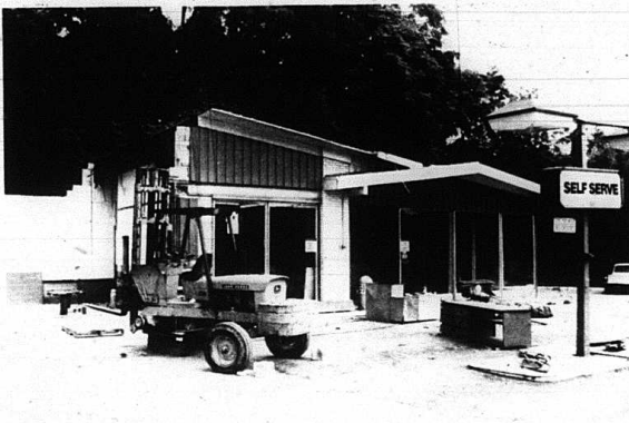
The Shell station near I-75 on U.S. 25 North is currently being remodeled by the owners, Carry Oil Co. of London. The station will be turned into a convenience store with self-service pumps. No word yet on when the station will re-open.
