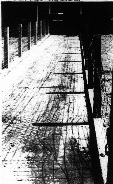
This concrete walk, from the barn to the milk shed, allows cows to get to the shed in orderly fashion and is easy to clean.
