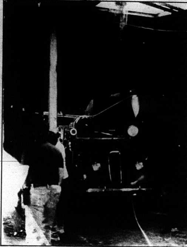
Workers rescued the city's oldest fire truck after the roof in the rear of Bryant Brothers Store collapsed, pinning the truck. Support beams, a bulldozer and a RECC truck were put to use in the effort.
