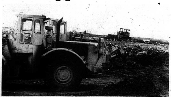
Site preparation is continuing for the new Rockcastle County High School. Construction is expected to begin about April 1 with the school being ready for the 1994 school year.
