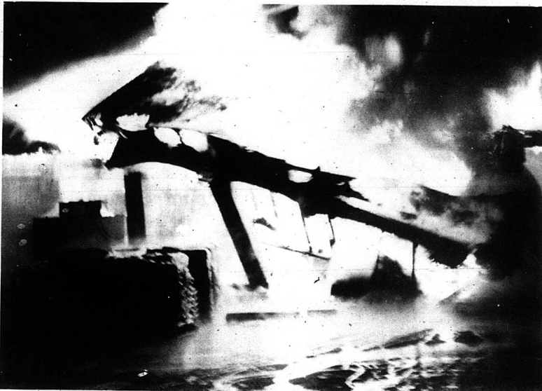
Fire completely destroyed Foodtown Supermarket early Friday morning but, through the efforts of the Mt. Vernon and Livingston Fire Departments, the Dollar General Store section of the building sustained only minor damage. In the
