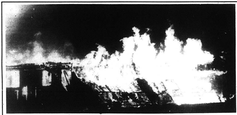
The home of Tom Miller on Negro Town Hill Rd. just north of Mt. Vernon was completely destroyed by fire very early Monday morning. The residence first caught fire on Sunday afternoon when the living room and kitchen were heavily damaged.
