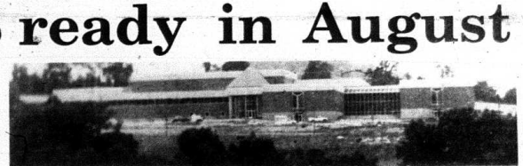
The new RCMS is located on the 461 By-Pass.
