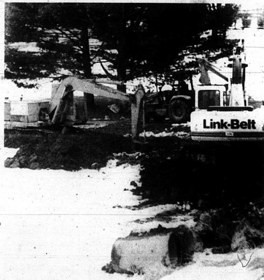
Work has begun on the Rockcastle County Industrial Park #2. Workers took advantage of the mild winter weather Tuesday to begin installing culverts on the park which is located on Hwy. 150, directly across from the current industrial park. One Richmond company has already said they would locate there.
