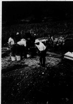
Jim Hammons, Eddie Hammond, Bill Dowell, Mike Prouty (Mobile), CL Furr (Mobile), and Kenton Parkey are seen with Honduran local help in the construction of the foundation of the Fields home.
