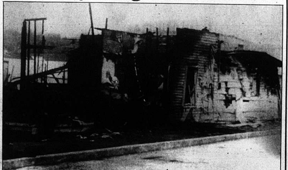
The home of Mr. and Mrs. Swannie Cummins on Crawford Street in Mt. Vernon was completely destroyed by fire early last Thursday morning. A trailer, sitting alongside the house, was damaged but city firemen managed to save it. The family lost everything in the fire.
