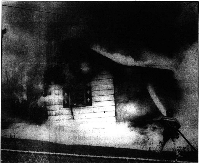
The home of Mrs. Shirley Smith, on Toddy Payne Road at Pine Hill, was destroyed by fire Tuesday. The structure was completely involved when firefighters from Mt. Vernon and
