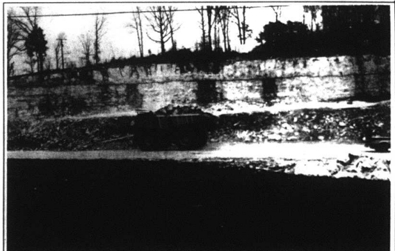
Taking it from here (top photo) and putting it there (bottom photo) has kept earth-moving crews busy now for several weeks. The work is taking place at the intersection of U.S. 25 and Richmond Street. A rock mountain across from McDonald's is being moved in the top photo and the rock from it is being used to fill the valley on U.S. 25 north of Wendy's. The U.S. 25 site will be the location for a new Wendy's when the site of the present Wendy's is taken to add two lanes to U.S. 25. Upon completion, there will reportedly be two southbound lanes, a turn lane and one northbound lane. The site across from McDonald's will be used as commercial lots.
