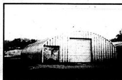
Metal Building with Concrete floor 48'x92'
