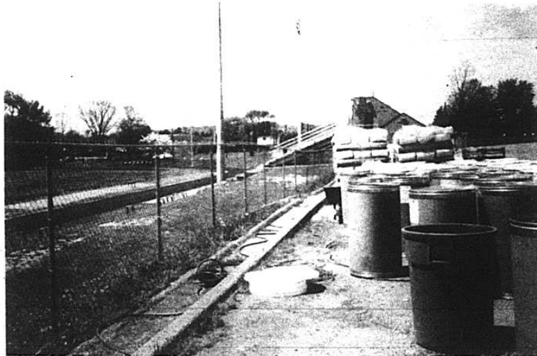
Over the week that it took to lay the new track surface, the parking lot was littered with large drums of packaged rubber. The track took only three days to complete, and two more days to paint.
