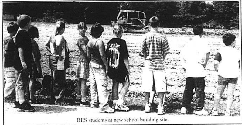
BES students at new school building site.
