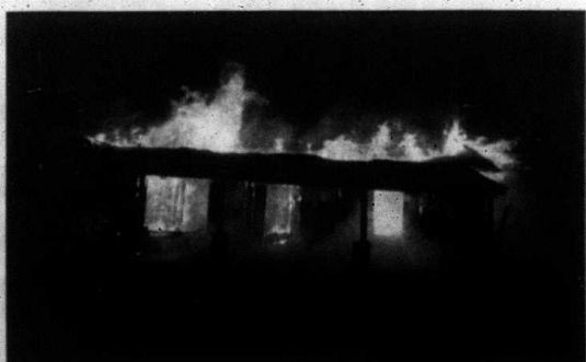
The home of Mike Alcorn on Barnett Road was destroyed by fire last week. When firefighters arrived, the structure was completely involved. Last Wednesday, a vacant home on Brindle Ridge was also completely destroyed by fire.
