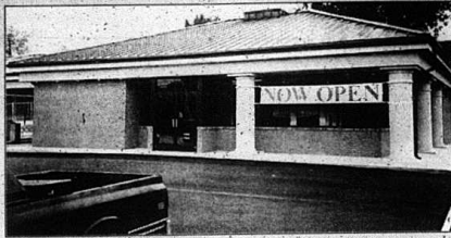
The new Berea National Bank of Mt. Vernon is located on Richmond Street next to the United State Post Office.
