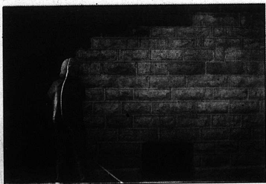
Sandblasting has begun on the outside of the gymnasium at the former Livingston School.
