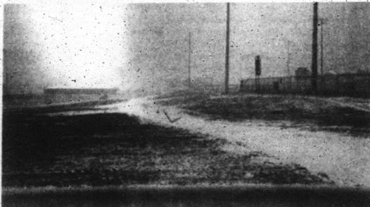
Snowfall and rain have contributed to delays on the new parking lot exit. Located at the far end of the parking lot, the exit will be for right-hand turns only. (photo by Brian Reynolds)
