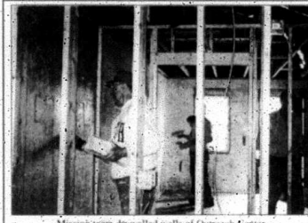
Mission team drywalled walls of Outreach Center
