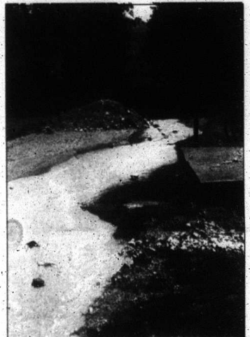
Sunday's heavy rains caused a lot of problems for residents of the Robert Ford Subdivision in Mt. Vernon. City maintenance supervisor Dennis McClure had to use a backhoe to clear the street from the rocks and debris that was swept into it. Shown above is the result of his clean-up and an exposed sewer line. McClure said that water washed away the covering over the sewer line. Residents on the street believe the water is coming from the Castle Ridge Subdivision, which is located on the hillside next to Liberty Drive. Mt. Vernon Mayor Karen King and one of the subdivision owners, John Clontz, said they were working this week to correct the problem.
