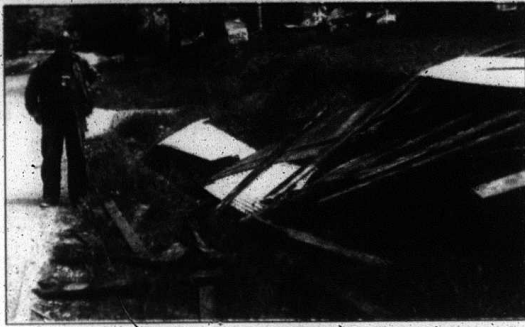
Darrell Cress, who lives on Wadd-Jones Road, stands besides part of a roof that was on his barn before a Sunday morning storm took most of it off. Several trees were uprooted and several buildings, mostly barns and outbuildings were damaged by the apparent small tornado.
