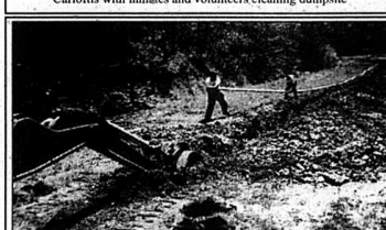
Waterline to homes under construction with inmate labor
