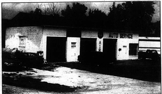
The Brodhead Volunteer Fire Department purchased the property of Danny Dillingham's on Hwy. 70 on Saturday for $45,500. Brodhead Rural Fire Chief Johnny Benge said that the garage and lot will be converted to a fire department substation for the western portion of the county. The new fire station will eventually lower insurance rates for residents in the area. Benge said the Rural Department already had a fire truck and that as soon as possible they would convert the building to a fire station. The fire department is soliciting and accepting donations to help pay for the property. For more information contact Benge at (606) 758-0206 or Brodhead Council member Everett Albright at (606) 758-9633. Donations can also be made at Citizens Bank in Brodhead and at B & L Grocery in Quail.
