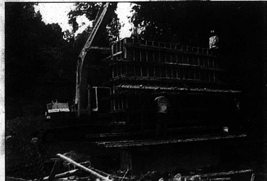
Work is continuing on the new bridge on Mullins Station Road. The bridge is scheduled to be complete sometime in August and currently residents are driving through the creek bed. N&N Contracting has the $155,000 bid on the project.
