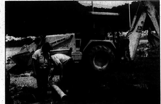
Mt. Vernon maintenance workers were busy this week fixing water lines and sewer lines in the city and out. The hot temperatures have made it difficult for people working outside, but when things tear up they must be fixed, according to the city's maintenance supervisor, Dennis McClure.
