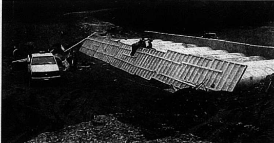
A low water ford is being constructed on the Ten Foot Hole Road near Livingston. The road connects U.S. 25 with Piney Branch Road. The Federal Emergency Agency is footing a lot of the cost for the bridge.
