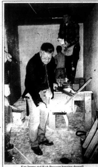
Ken Ipema and Rich Brouwer hanging drywall.
