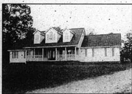
New House Completed
