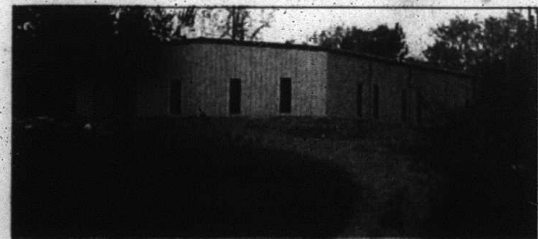
The above building, located on the Hwy. 461 by-pass, which will house an Adult Day Care Center, is in the process of being built. The owners of the property say they will have activities for seniors and will provide meals and that RTCC will provide transportation to the center, once in operation. The facility is scheduled to open sometime this summer.
