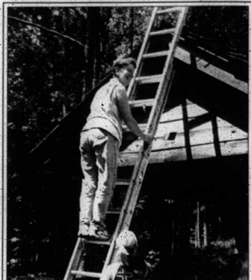
Pam Van Riessen varnishing the covered bridge.
