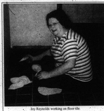
Joy Reynolds working on floor tile
