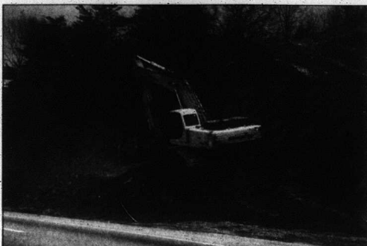
Construction at Conway and at the Rockcastle River is scheduled to be complete by November. Shown above is construction work being done at Conway on Wednesday morning.
