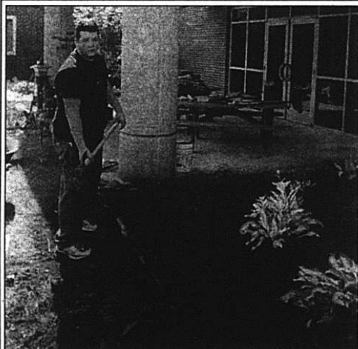
Brandon Lamb busy digging trenches for the new landscape.
