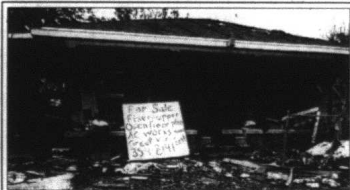
Some people still can find humor in all this tragedy. One sign says "For Sale - Fixer Upper - Open Floor Plan - AC works - Great View"
