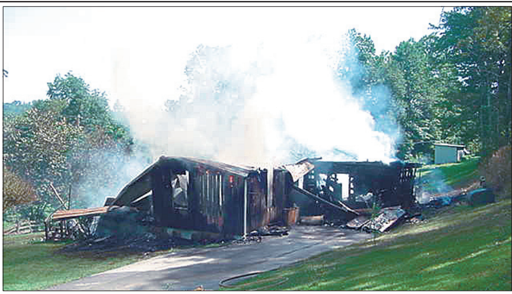
The home of Randy and Michelle McClure at Buffalo was completely destroyed by fire on Wednesday morning. Members of the Mt. Vernon Volunteer Fire Department, Brindle Ridge Fire Department and firemen from other departments responded to the 10:30 a.m. fire. McClure said his wife told him the fire started in the cabinet section of the kitchen. The McClures have two children and lost everything in the fire, including some items that Mrs. McClure had managed to throw out of the home after she realized it was on fire.
