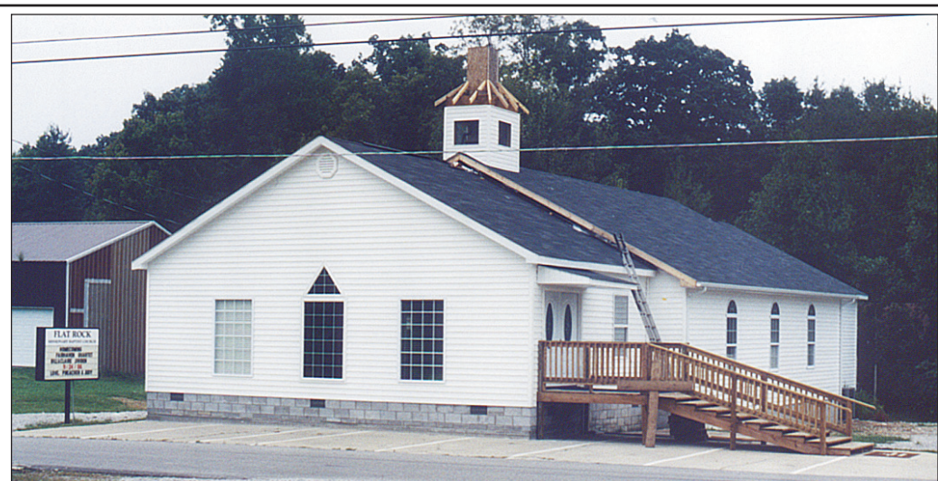
Renovation is complete on the Flat Rock Baptist Church after a June 4th electrical fire damaged the building. Flat Rock Baptist, which is located at Maple Grove, is probably Rockcastle County's oldest Baptist Church being established 122 years ago. Church members have held services in their renovated building the past two weeks and have scheduled a homecoming and dedication service for Sunday, September 24th. The homecoming starts at 11 a.m. and the dedication service begins at 2:30 p.m.
