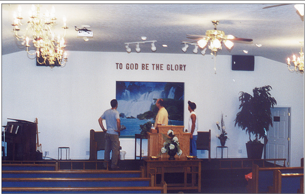
Mark Laswell, left, Dr. Larry Burton, pastor of Flat Rock Baptist Church and Donald Brown look over some of the work done on the church after a June fire. Dedication services for the renovated church will be held Sunday at 2:30. Homecoming starts at 11:00 and Laswell will be ordained into the ministry in a 3:30 ordination service. Laswell, Burton and Brown are among many volunteers who have helped work on the church since the fire. The renovation costs approximately $78,000. Flat Rock Baptist is located on Maple Grove Road.
