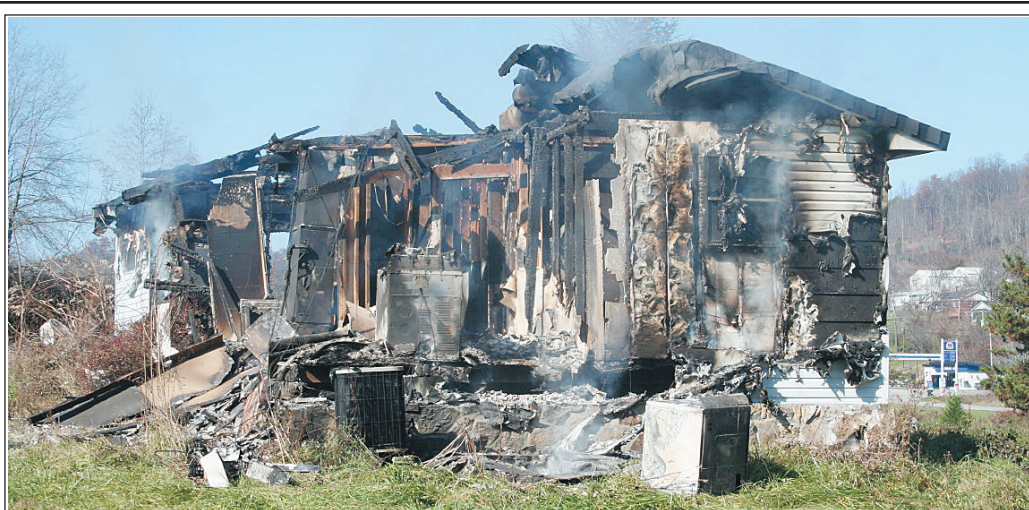
A vacant mobile home owned by Charles and Kathy Brock of Burr was destroyed by fire last Wednesday morning. Mt. Vernon firefighters got the call around 5:15 a.m. Public Affairs officer Steve Griffin said the mobile home was completely engulfed when firefighters got the call. The mobile home was still burning on Thursday and officials think the smoke from the fire, combined with the heavy fog on Thursday morning, may have caused "smog". It was the second trailer of the week in the Burr area to burn. A doublewide mobile home was destroyed by fire on Monday morning. Both mobile homes were located near the exit 59 ramp where seven wrecks involving 20 vehicles occurred Thursday morning.
