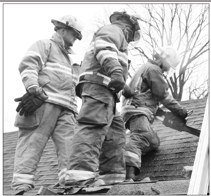
John Dyehouse instructs Luther Allen and Chris Kerns the proper techniques of vertical ventilation. Vertical ventilation is achieved when the smoke, fire, and super heated gases can escape through an opening directly above the seat of the fire. This technique aids in clearing the smoke for interior fire attack crew to see and extinguish the fire.
