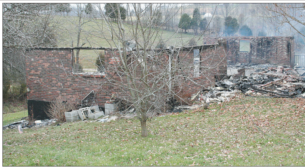
The vacant house of James and Judy Kidwell on Doc Adams Road (Old Hwy. 461) was completely destroyed by fire early Saturday morning. Mt. Vernon firefighters got the call around 6 a.m. and when they arrived a few minutes later, the house was completely involved. Fire Chief Gary Hansel said the fire was obviously set and an arson investigator from the Kentucky State Police was investigating the fire.
