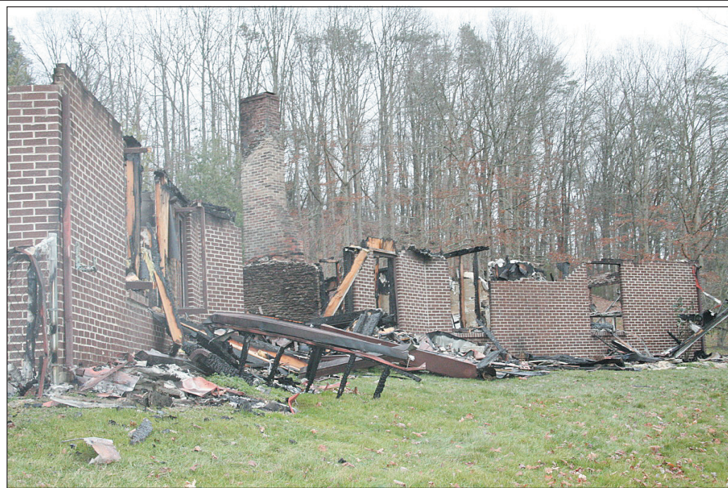
The home of former Rockcastle County Deputy Sheriff Kenny Holt was completely destroyed by fire Saturday night at Fairview. Holt said that heat tape on water lines under the porch caused the fire. Brindle Ridge, Mt. Vernon and Brodhead departments all responded to the call around 10:30 p.m.
