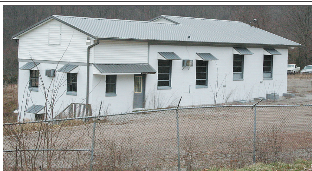
The Mt. Vernon Volunteer Fire Department and emergency vehicles used by the county's CSEPP program will be housed in a new 7,200 square foot building on the former Rockcastle County road department garage property on Old U.S. 25 in Mt. Vernon. The old building above will be used for training and other needs.
