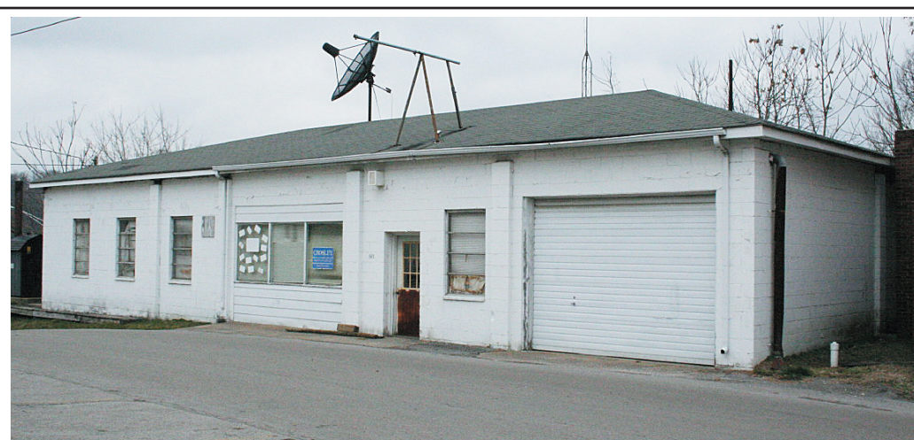
The former Eaton Electronics' building on Spring Street in Mt. Vernon will be converted into a cafe by RTEC in the next few months.
