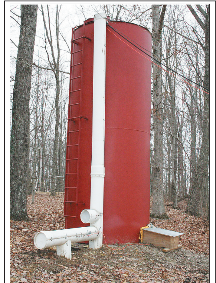
One 3,000 gallon water storage tank located at cleftRock is already operational and has been used to help fight fires in the area.
