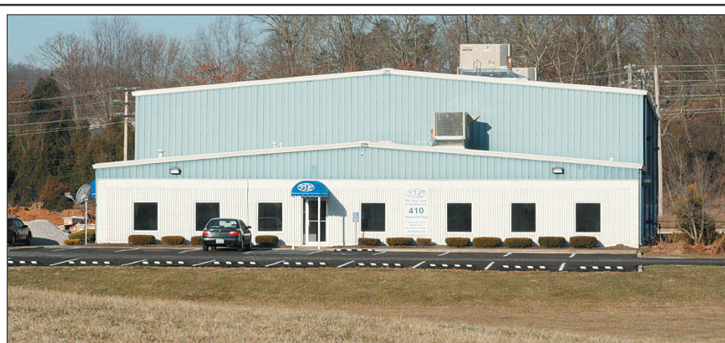
FPL Door Locks and Hardware could open in Rockcastle Industrial Park #1 as early as August.
