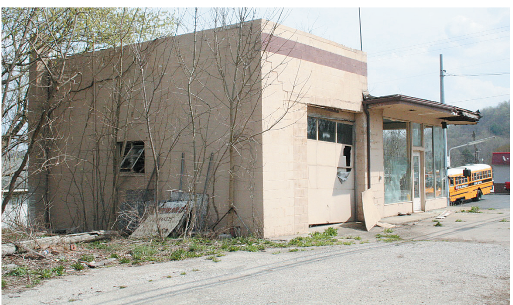
A Main Street grant proposal calls for the renovation of the above building, which would be used for a Farmer's Market. The building is owned by Johnny St. Clair and located at the corner of Richmond Street and Highway 150 in Mt. Vernon.
