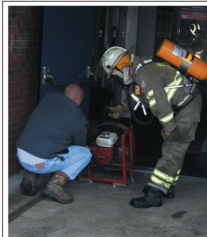
Mt. Vernon firefighters Jason Hansel and Jackie Weaver placed an exhaust fan at the back entrance to the middle school on Friday morning to help clear smoke out of the building heavily damaged by an early morning fire.
