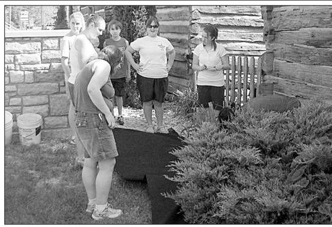
Band members lay garden fabric for the stone near the cabins.
