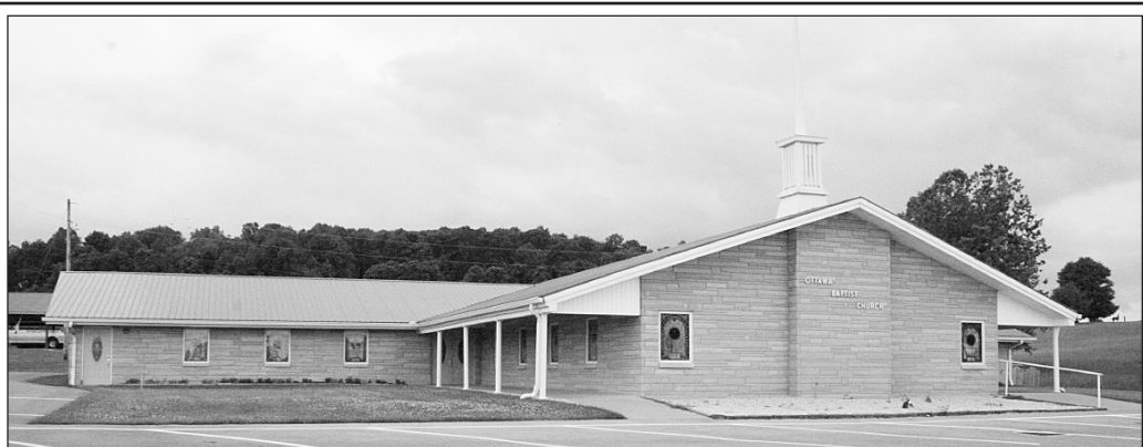
Services at Ottawa Baptist Church have been held in the same building since 1963 with many improvements and expansions through the years.
