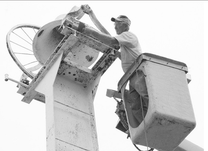
Longtime active Ottawa Baptist church member Paul Cash was busy Saturday refurbishing the church's bell, scraping the old paint and giving the bell and tower a new coat of paint.
