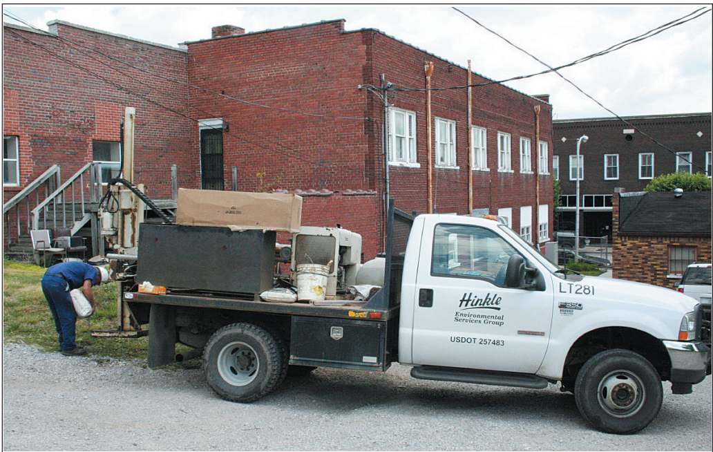
Johnny Burchell of Hinkle Environmental Services was busy Tuesday core drilling behind Dr. John Parsons' office on Main Street in Mt. Vernon. The state's environmental agency is attempting to find the source of a gas smell which has been getting into Parsons' office for the past several years. Samples from the core drilling have been sent to Frankfort. Parsons' office was closed Monday and Tuesday because of gas smell.
