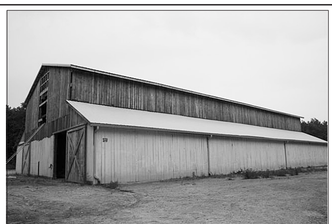
This 16,000 sq. ft. horse barn includes stalls for horses and animals, an indoor archery range, rock climbing wall and repelling station.
