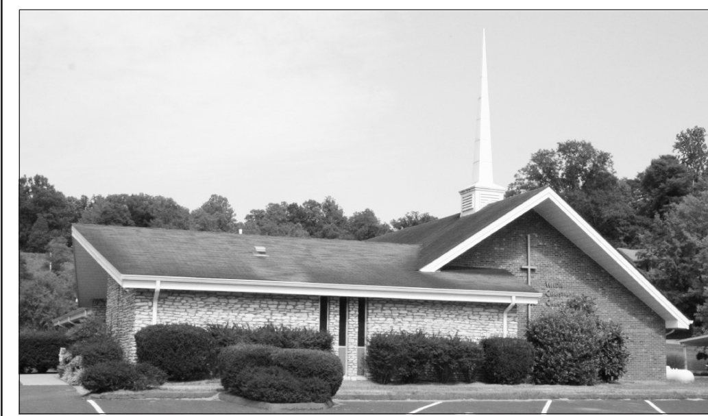
The current Wildie Christian Church building was built in 1975 and is located on Wildie Road.
