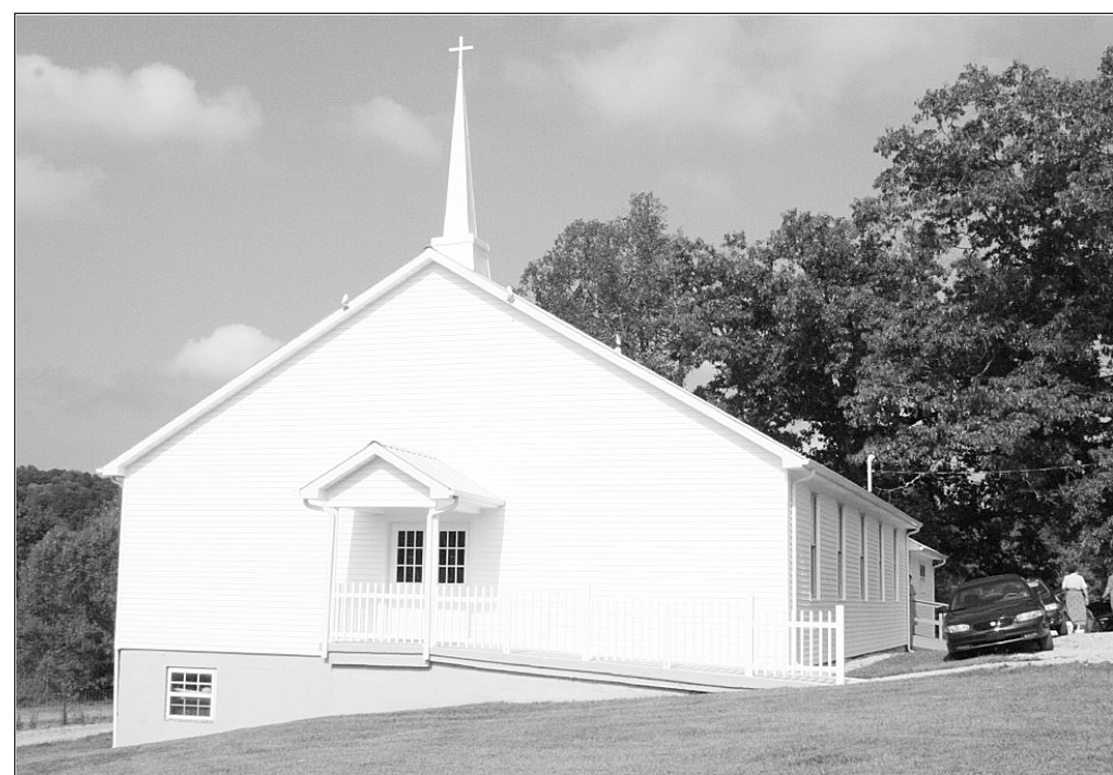
Roundstone Missionary Baptist Church recently underwent a $75,000 renovation project, which completely remodeled the original structure built in the early 1940's. (Roundstone Baptist Church photos by Richard Anderkin).
