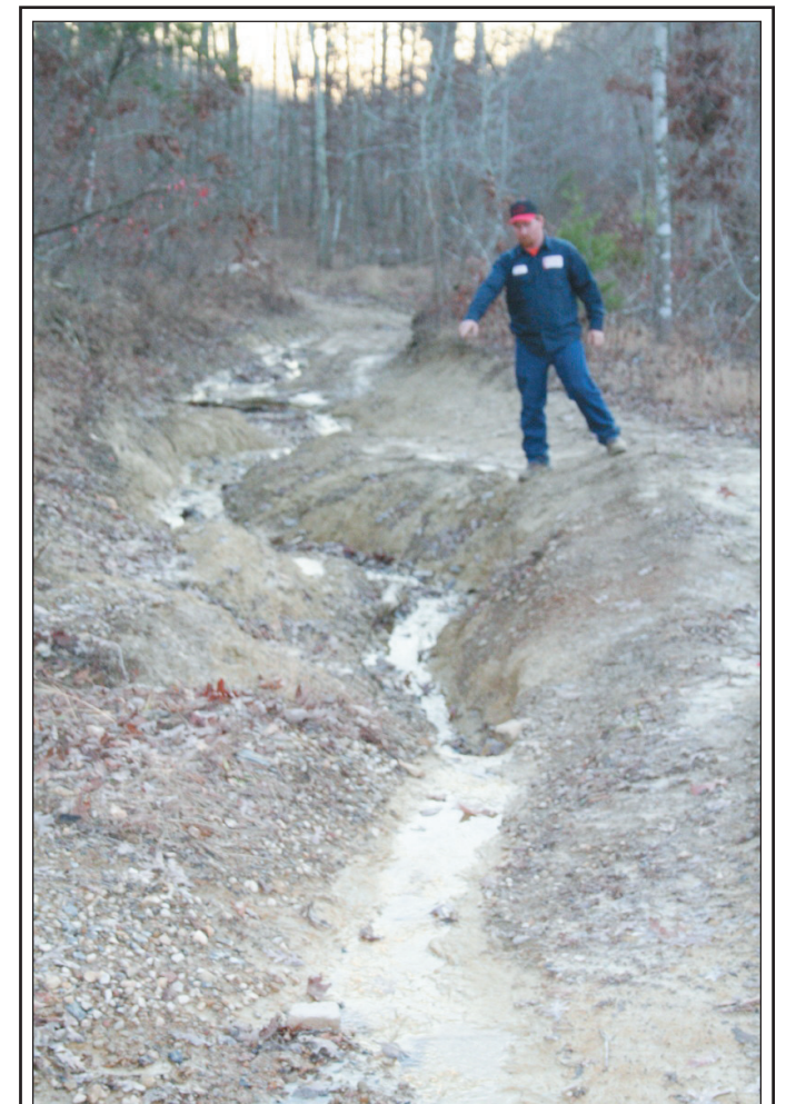
Brindle Ridge fireman Scott Powell points to the place in the Old Gabbard Road, where Leon Farris's vehicle became stuck last Thursday morning. The photo shows how bad a shape the county road is in and why Farris couldn't travel along it. He did not remember turning onto the road off of Lambert Road Thursday morning.
