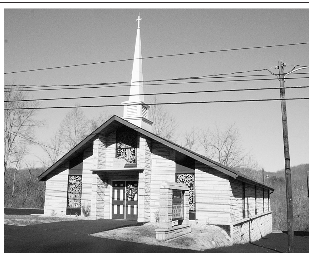
The new Livingston Pentecostal Church is located on U.S. 25, just north of Livingston. Construction on the new church began in 1974 and the dedication for the new church was held in 1975.
